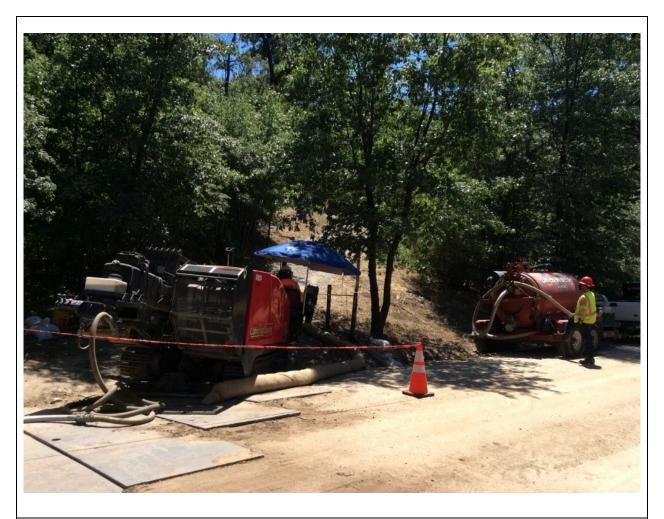
**Photo 5:** Site-specific erosion control BMPs were used under the directional drill on Los Huecos Road (C 440) to contain drill mud that may result from the activity in accordance with the SWPPP and APM HYD-09.
