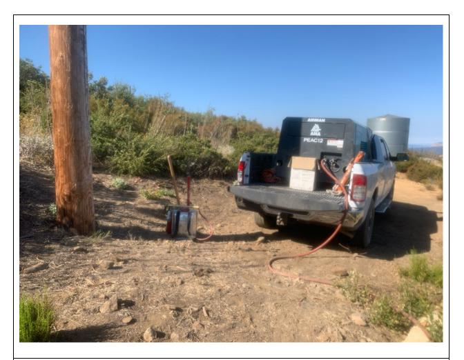
**Photo 4:** A running air compressor at Pole P258572 (C 79B) had at least 5 feet of clearance from combustible material on all sides and a full set of fire tools (5-gallon backpack pump, round point shovel, Pulaski, and 2A10BC fire extinguisher) within 50 feet in accordance with the CFPPP Fire Prevention Matrix for combustion engine use off USFS land with an Elevated FPI.
