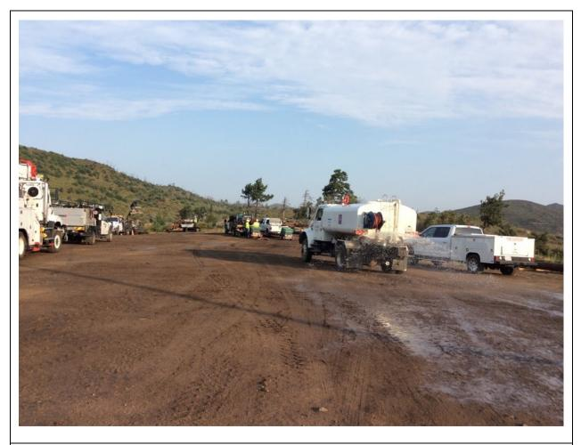
**Photo 1:** A water tender was observed applying water to the surface at Shrine Camp Staging Yard (C 440) before and during helicopter activities to minimize dust emissions from rotor wash in accordance with APM AIR-02 and the Aviation Safety Plan (MM PHS-5).
